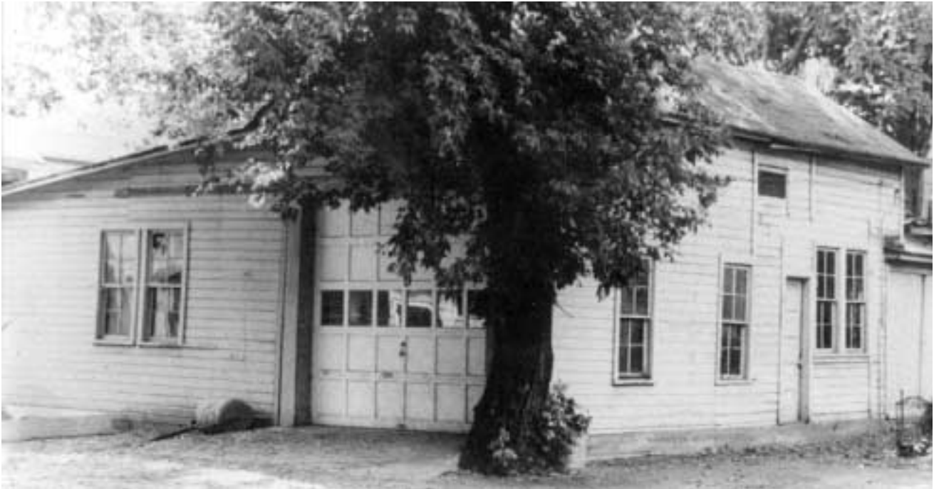
Miller's Garage was located behind the Miller home at 607 South Blackstone Street
